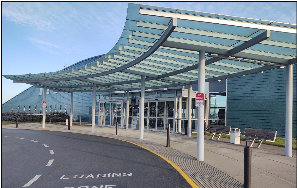
Figure 1-8 Passenger Terminal Southwest Oregon Regional Airport
